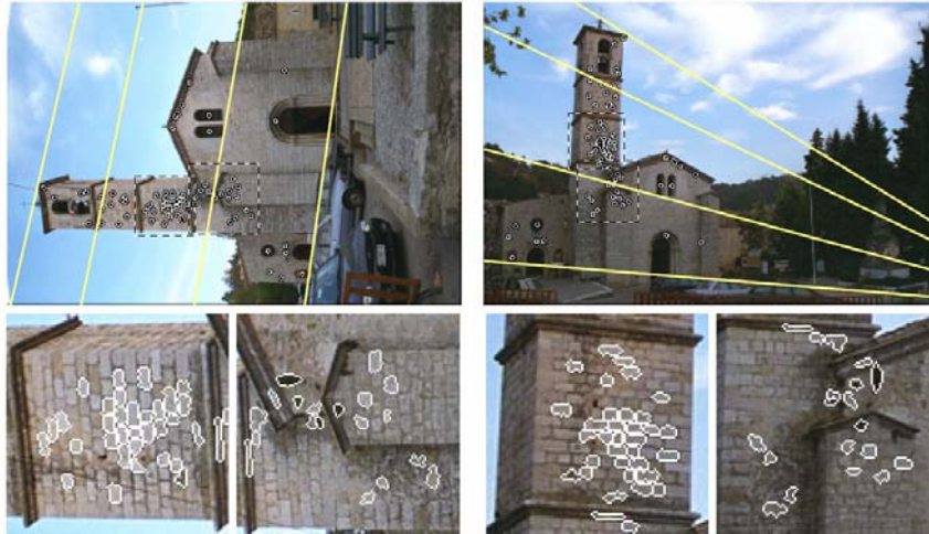
Figure 2: VALBONNE: Estimated epipolar geometry and points associated to the matched regions are shown in the first row. Cutouts in the second row show matched bricks.
