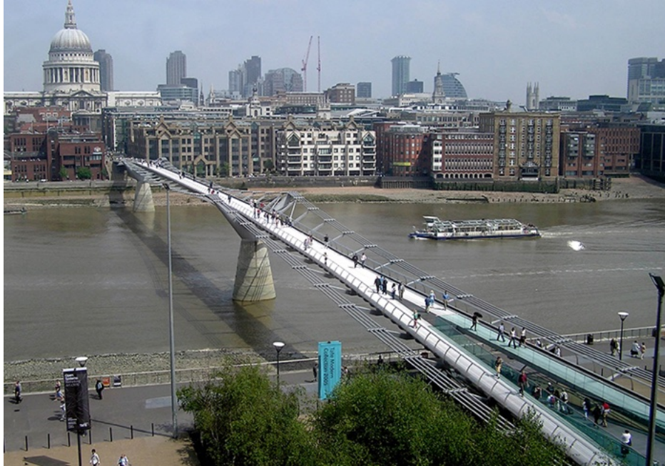
Figure 15.33 Initially when people crossed the London Millennium Footbridge, they experienced a swaying motion. People continuing to cross reinforced the oscillation’s amplitude, thereby increasing the problematic swaying. (credit: Adrian Pingstone/Wikimedia Commons)
