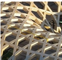
Figure 4: Timber construction for the Yeosu Golf Club by Shigeru Ban; CAD/CAM by designtoproduction . The beams are not geodesics and manufacturing thus requires CNC machining. We address the design of 3-patterns of geodesics and so contribute to their simplified manufacturing.
